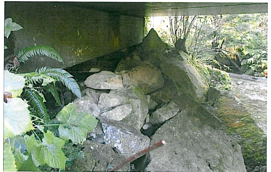
CK-2277 Left Abutment
