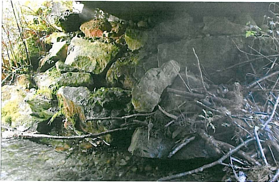
CK-2277 Right Abutment
